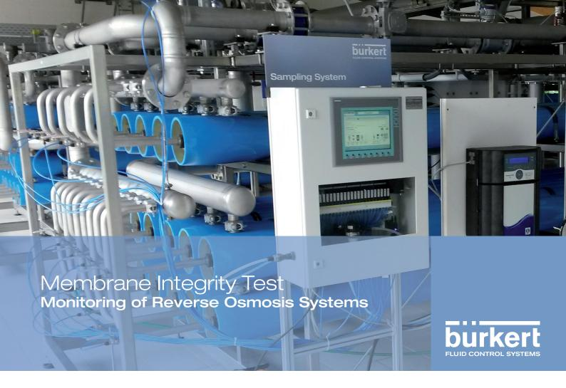
The sampling system uses sensors to measure the water quality of individual pressure pipes. The water sample is extracted through valves and conveyed automatically to the sensors. Parameters such as conductivity, turbidity and chlorine are measured at this point. The measured values are subsequently compared with limit values and logged. Afterwards the data is available for further evaluations.
